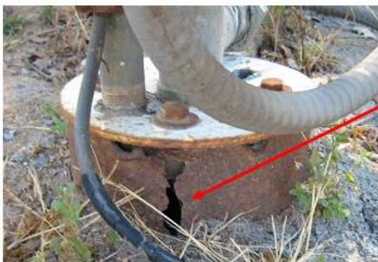
A cracked well casing may allow surface water and contaminants into your well. One of the most common water quality issues associated with a cracked well casing is the presence of coliform bacteria. Other chemicals can also be introduced into the well through the cracked casing. Consult a water quality professional, such as a licensed well driller, to repair or replace the cracked casing.
