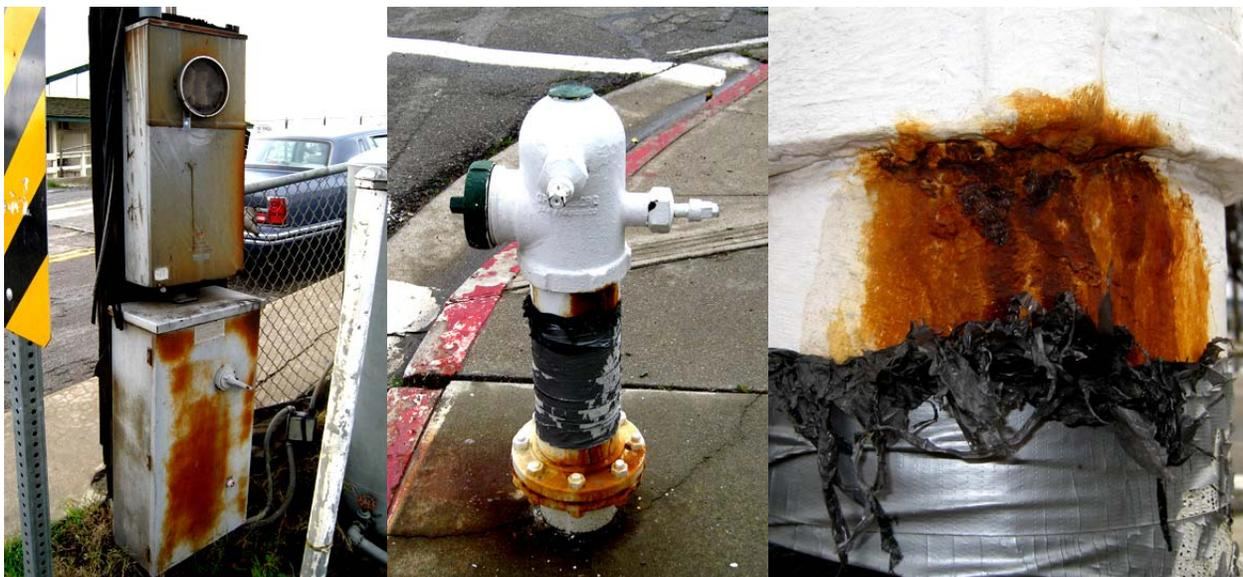
Abandoned switch meter box for pump, and an unused corroded fire hydrant in the business district
